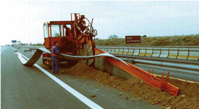
Figure 33: Installation of composite drainage as road shoulder drain
